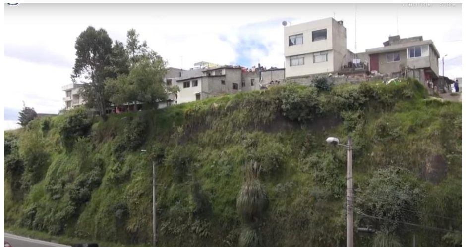
Houses in danger
