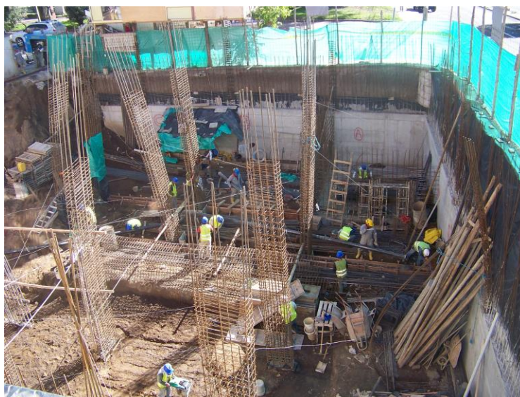
Construction site early December
