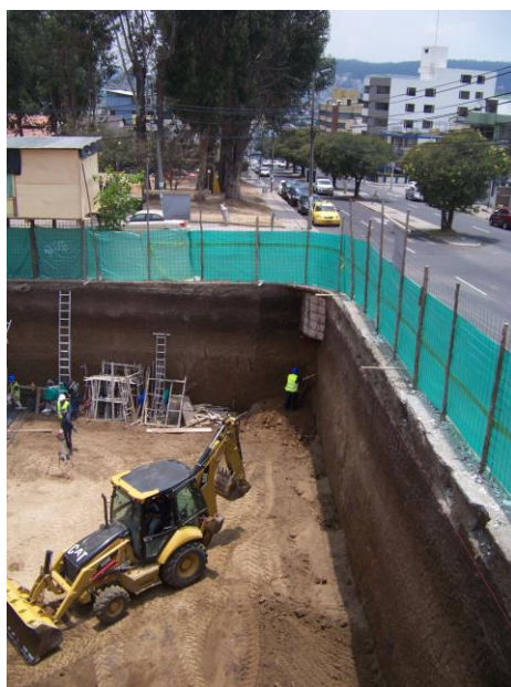
Construction site October 1 viewed from our balcony
