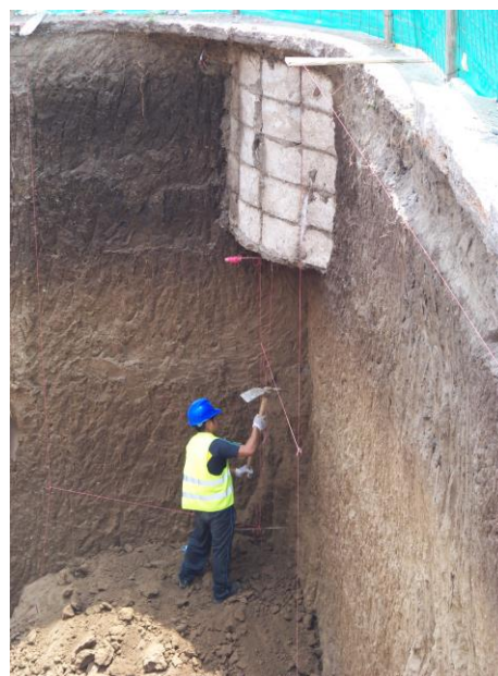
The rope is the guideline to make the cut straight.
